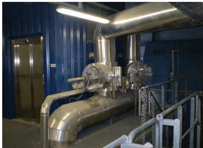
Obr. 4 - HP Steam Header
